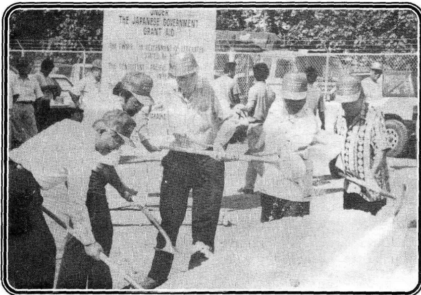
UPGRADING POHNPEI POWER PLANT - The Nanpohnmal Power Plant will be upgraded after the ground breaking ceremony held, April 12 which will provide an additional five mega watts of power. The project is expected to be completed in 11 months and will cost 8.5 million U.S. dollars. Above are the officials representing the Governments of both the FSM and Japan breaking the ground of the project.
